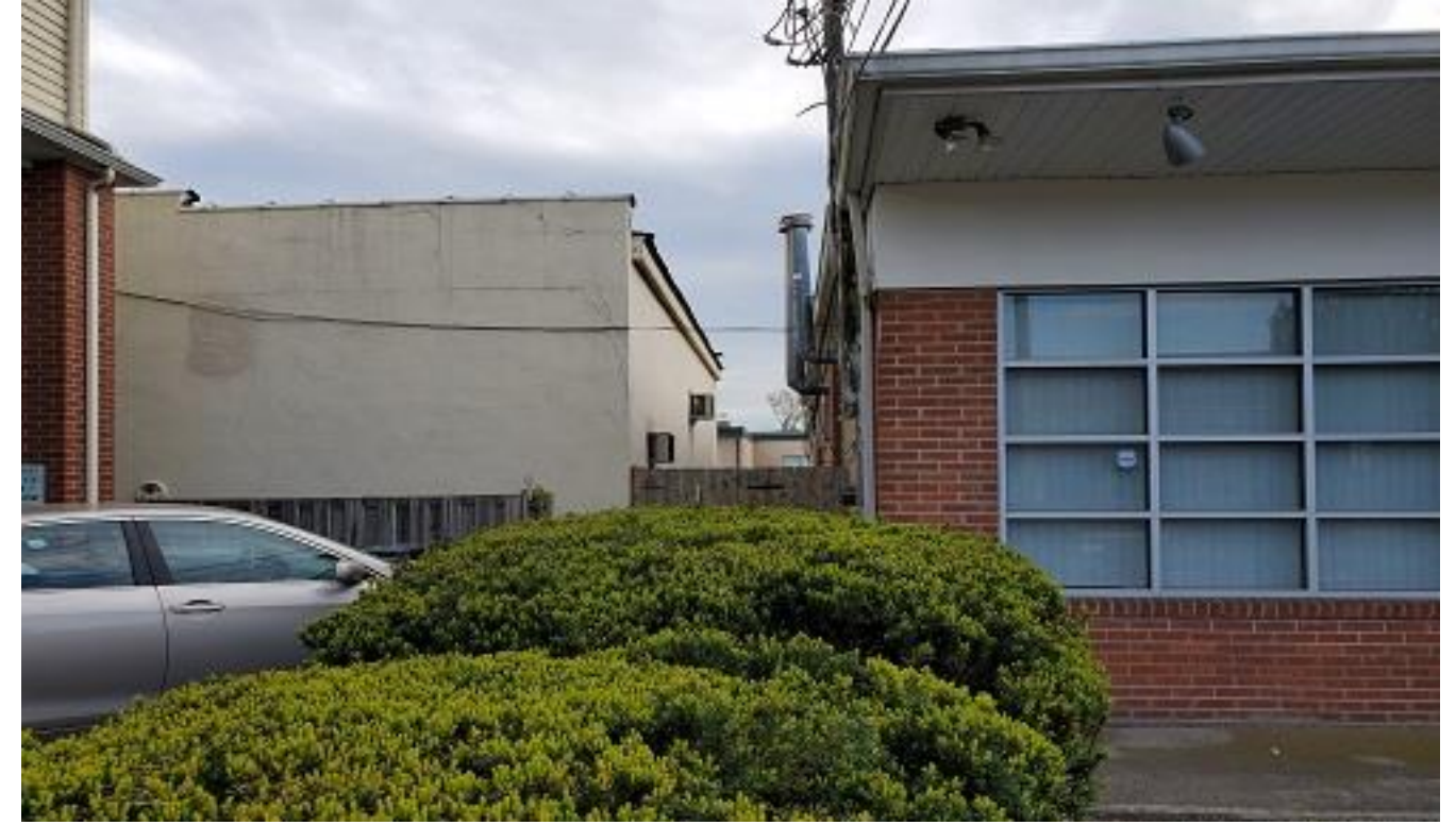
Image 3. View toward rear of subject building and east-facing side.
