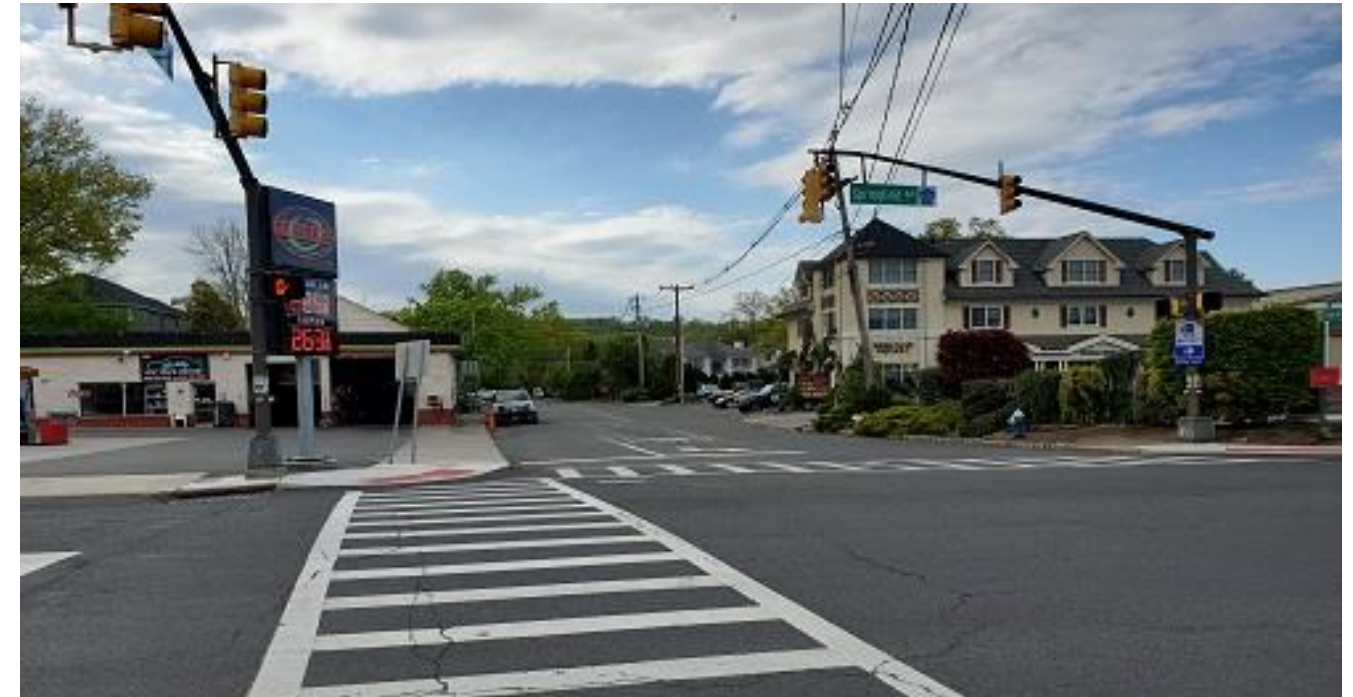
Image 9. Panning right from prior photo, commercial uses built close to street edge of Plainfield Ave, north of Springfield Ave, including 3-story structure and within retail center.
