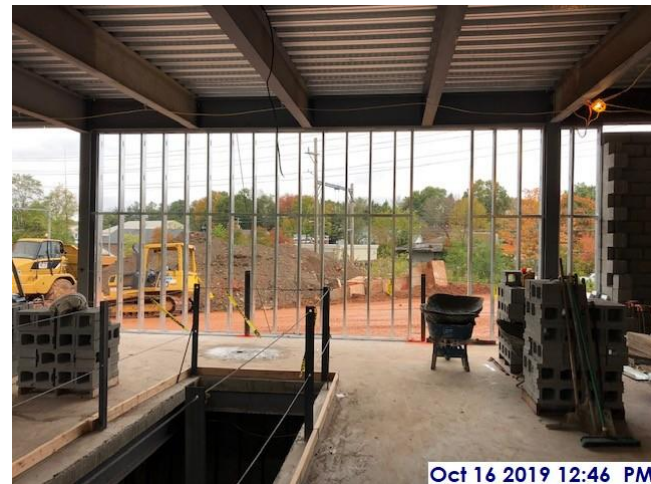
Start of 1 st floor exterior framing in police area
