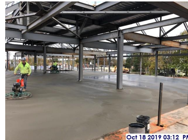
Finishing 2 nd floor slab on deck concrete, center sector
