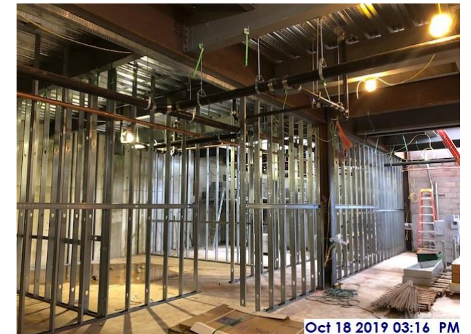
Interior framing for basement archive & storage areas
