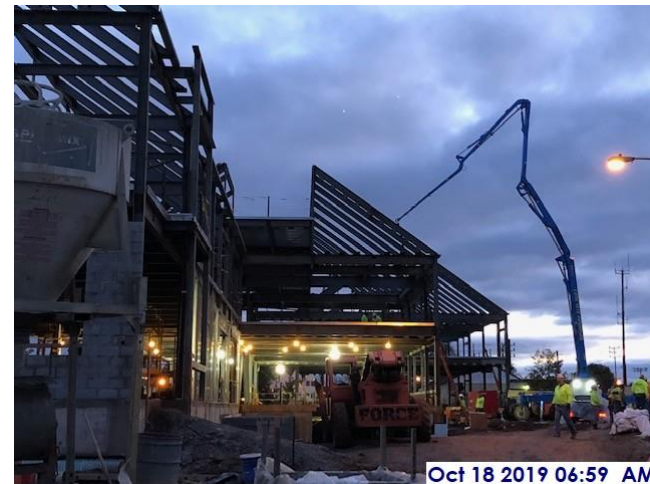
Concrete pump truck for slabs on deck, center sector
