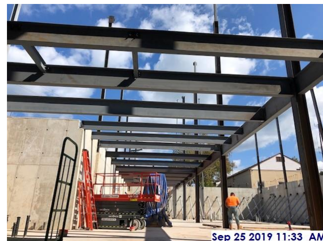
First beams set, east sector
