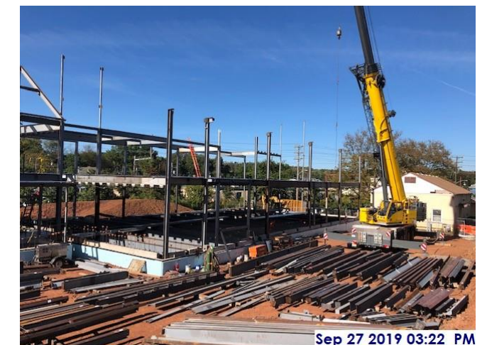
East sector steel erection progress
