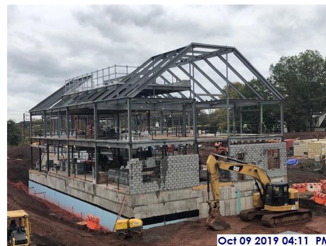
Block wall installation, west sector
