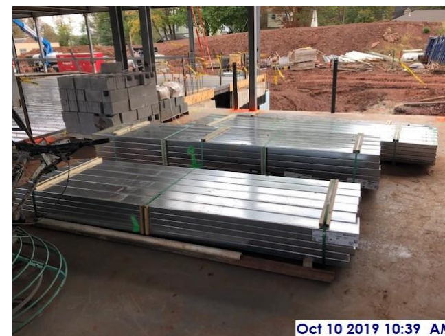
First delivery of metal framing
