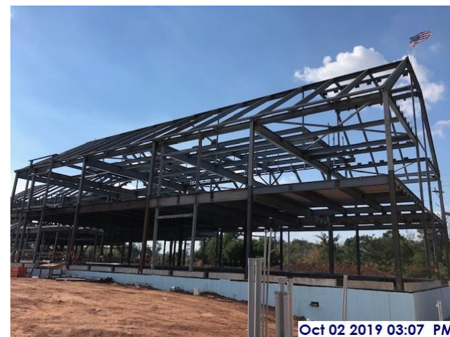
East sector steel erection substantially complete
