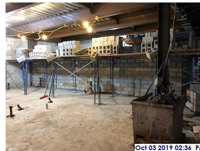
Masonry block work at Police Archives
