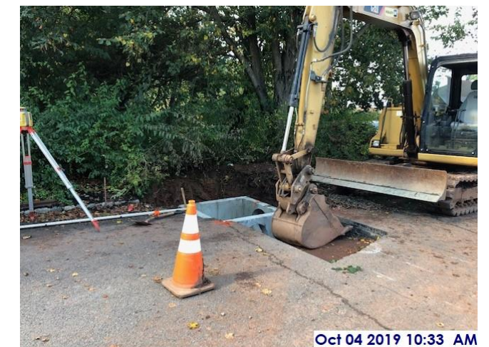
Storm inlet installation, Berkeley Ave.
