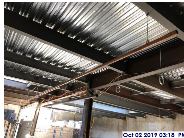
Plumbing line installation, west sector basement
