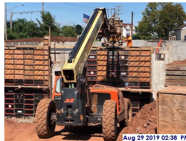
Pouring final section of foundation wall at access ramp
