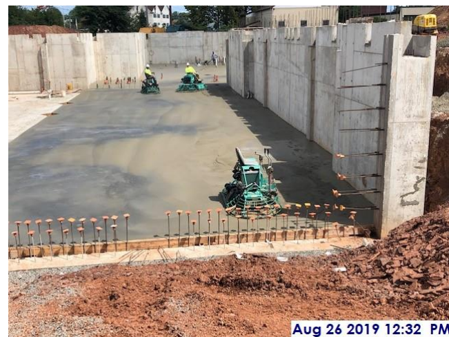
Finishing slab on grade, center/south sector
