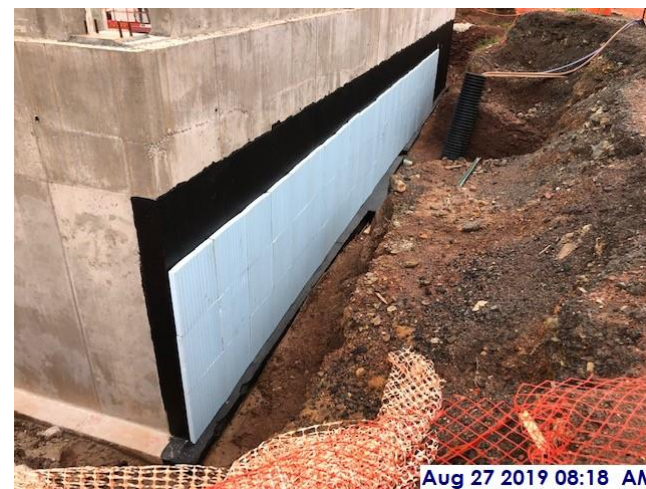
Foundation damp proofing & insulation board, west sector
