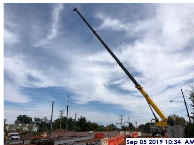
First steel columns placed, west sector
