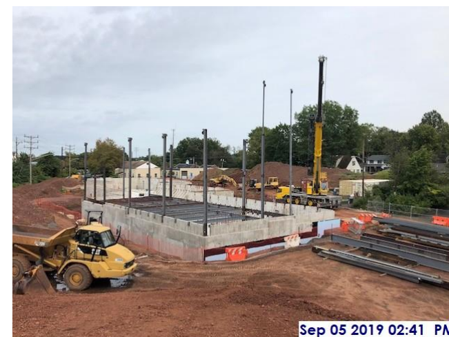
End of first day of steel erection, view from northwest
