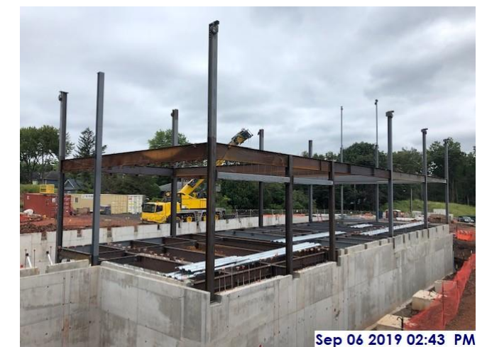
End of second day of steel erection, view from southwest
