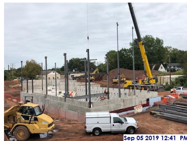
First steel beams placed, west sector
