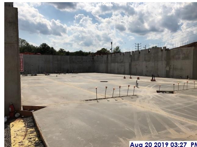
Slab on grade finished, west sector
