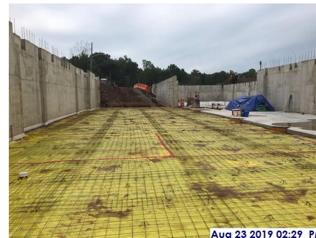
Prep for slab, center/south sector
