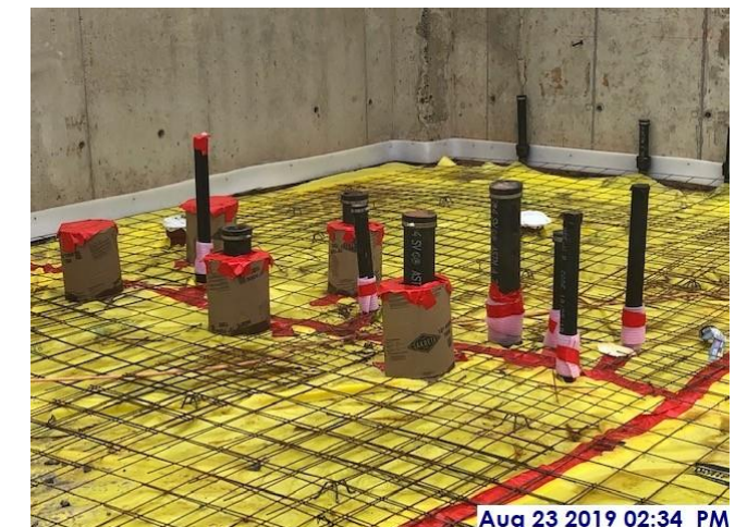
Sleeves for floor drains and cleanouts
