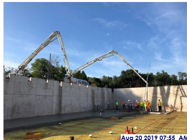
Pouring slab on grade, west sector
