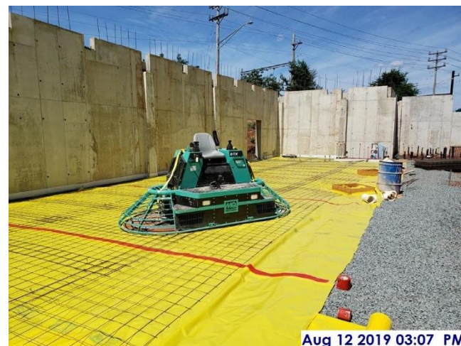
Vapor barrier & mesh for slab, center sector (north)
