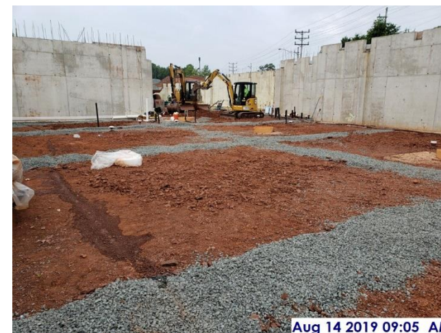
Under slab drainage, east sector
