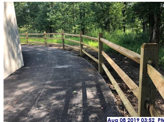
Split rail fence installed behind salt dome
