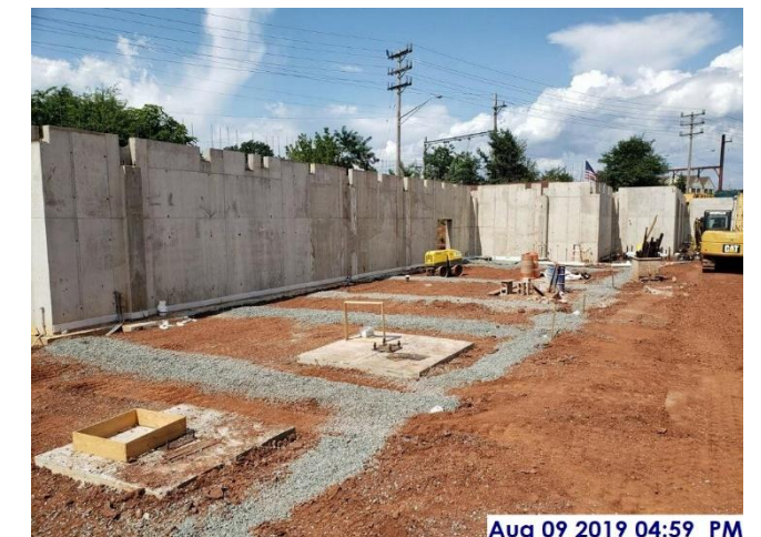
Under slab drainage, center sector
