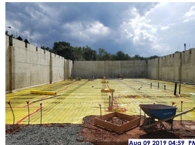
Vapor barrier & mesh, west sector
