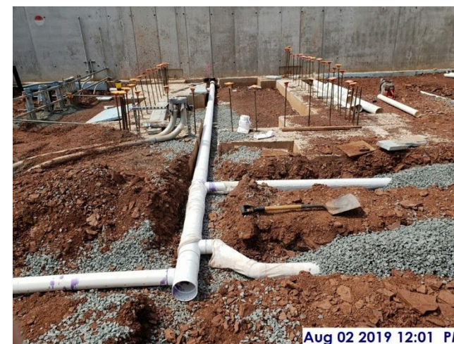
Under slab drainage, west sector
