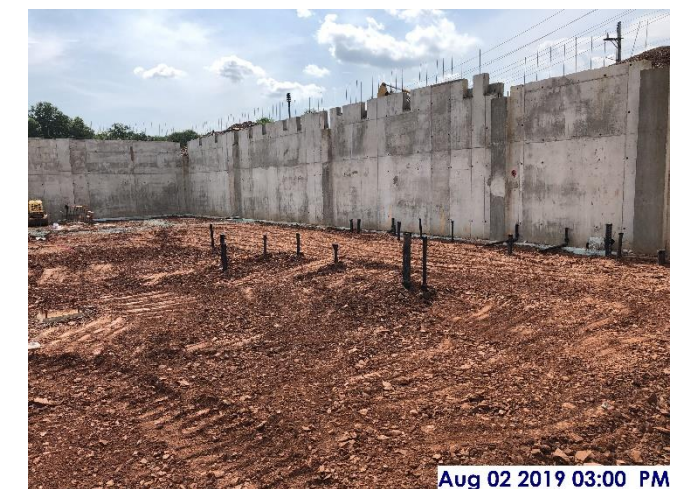
Backfill & compaction, west sector
