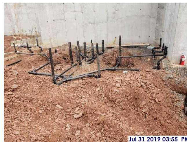
Underground plumbing, center sector
