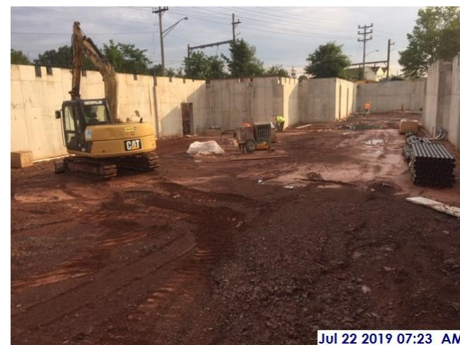
Prep for underground plumbing
