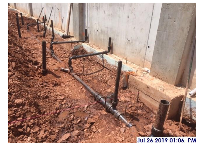
Underground plumbing risers
