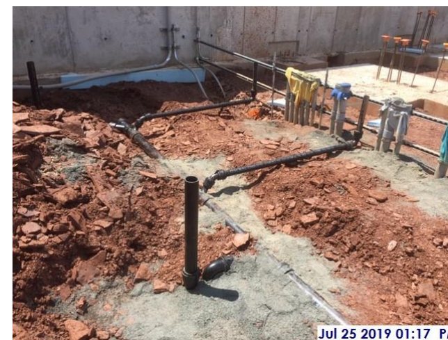
Backfill for underground plumbing
