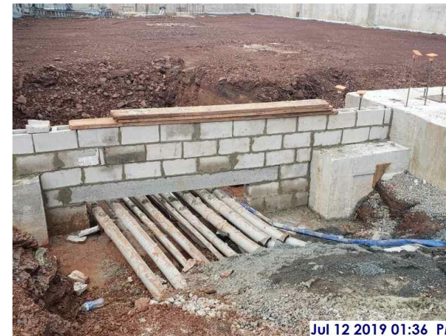
Precast lintel and CMU block at footing line
