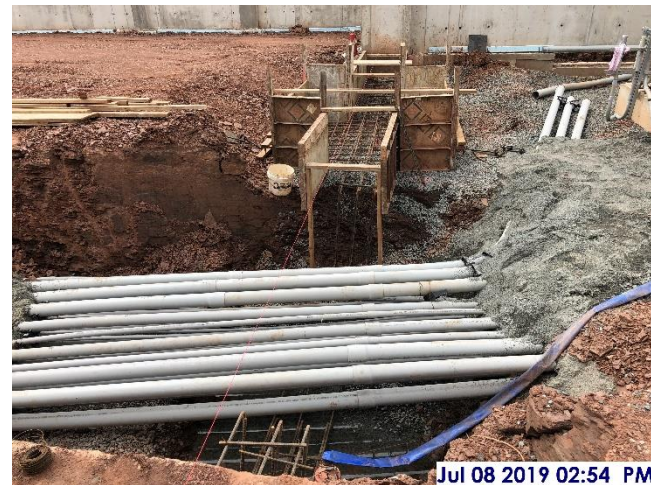
Form work and rebar for interior footing
