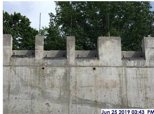
Leveling plates set at foundation walls, center sector
