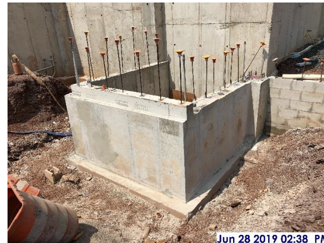
Elevator pit rubbed down in preparation for waterproofing
