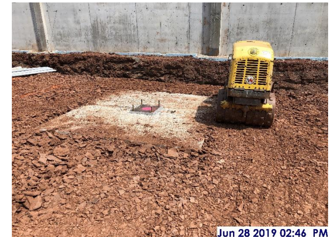
Pier footing C4 backfilled and compacted
