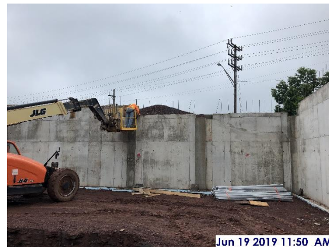
Stripping Beam Pockets
