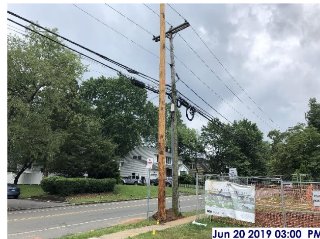
New Utility Pole Set by Verizon, Park Avenue
