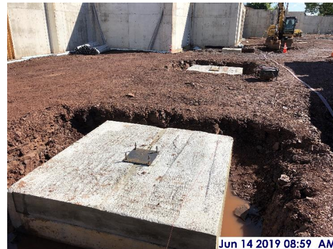
Pier footings with anchor bolts & base plate, west sector
