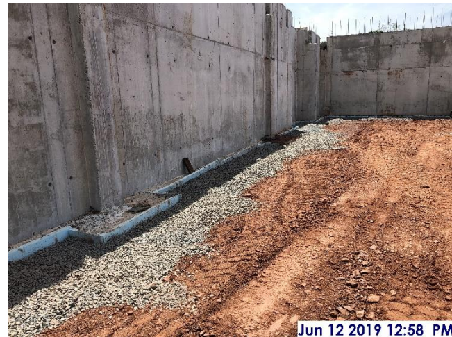
Stone backfill at footings, east sector
