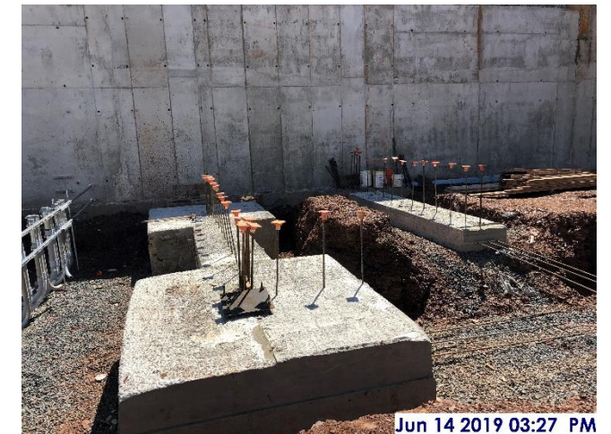
Stair #1 footings, west sector
