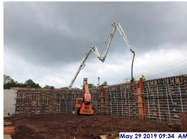
Pumping concrete for north wall, west sector
