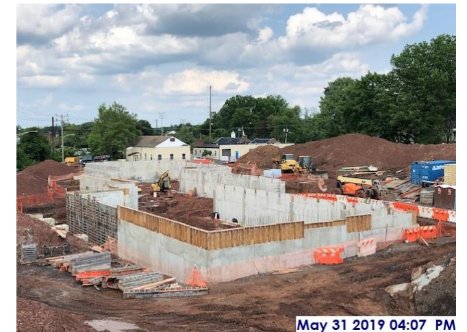
Foundation walls substantially complete
