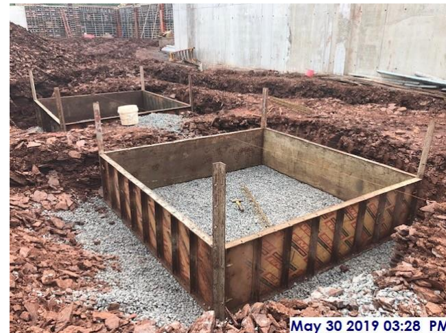
Form work & stone for interior pier footings, center sector
