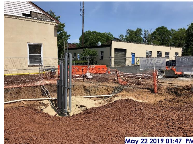
Backfill for electrical conduits at transformer location
