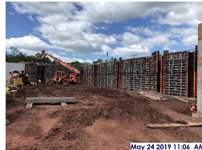
Closing up form work for foundation walls, west sector
