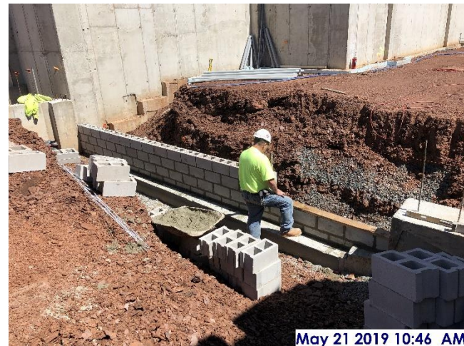
Building masonry wall
