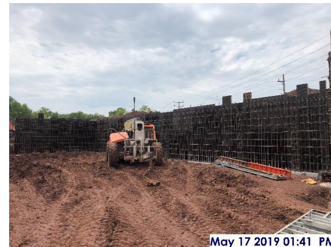
Form work for foundation walls, west sector
