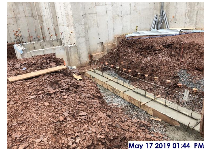
Footing poured between east and west sectors
