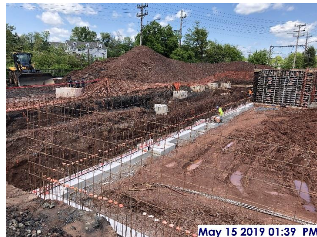
Rebar for foundation walls, west sector
