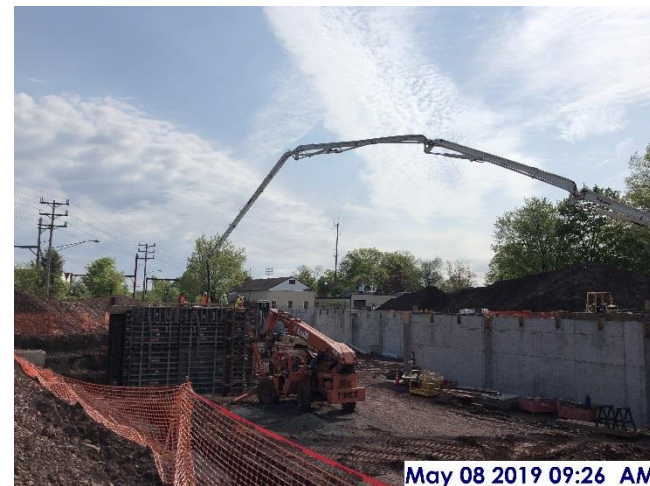
Pumping concrete, center sector
