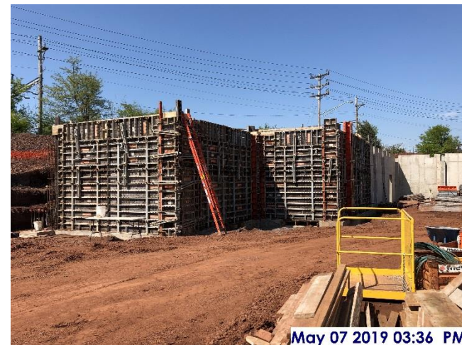
Form work closed for pouring concrete, center sector
