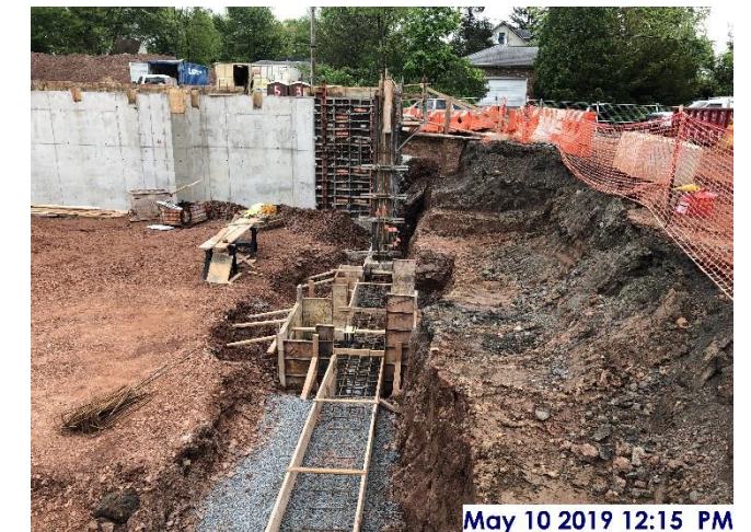
Form work for footings, west sector
