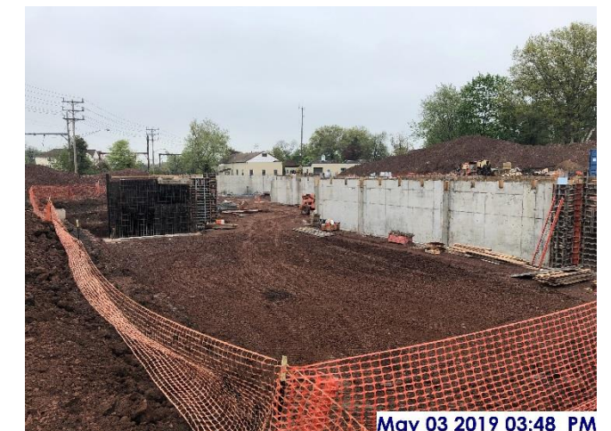
Excavation in building footprint substantially complete
