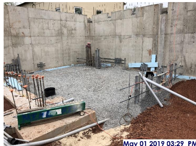
Backfill at main electrical room
