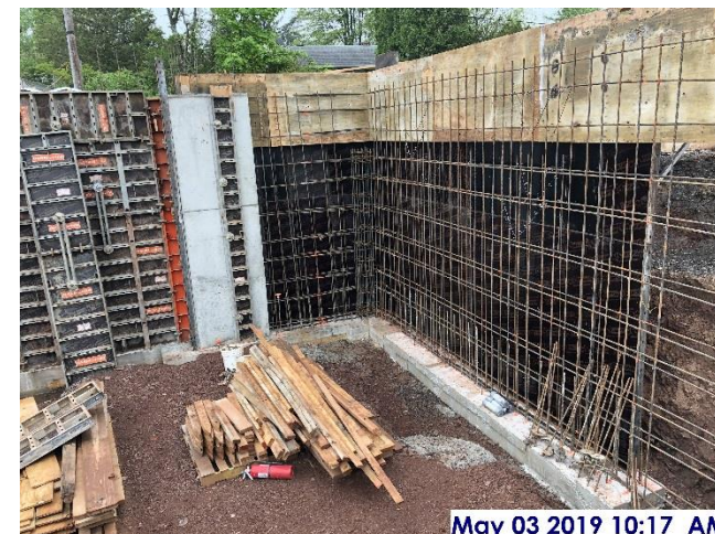
Rebar and form work for foundation wall, west sector
