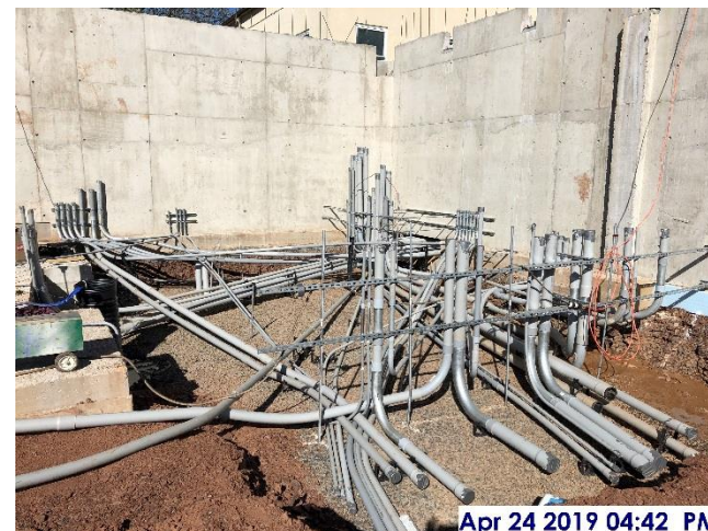
Apr 24 2019 04:42 PM Underground conduit for main electrical room
