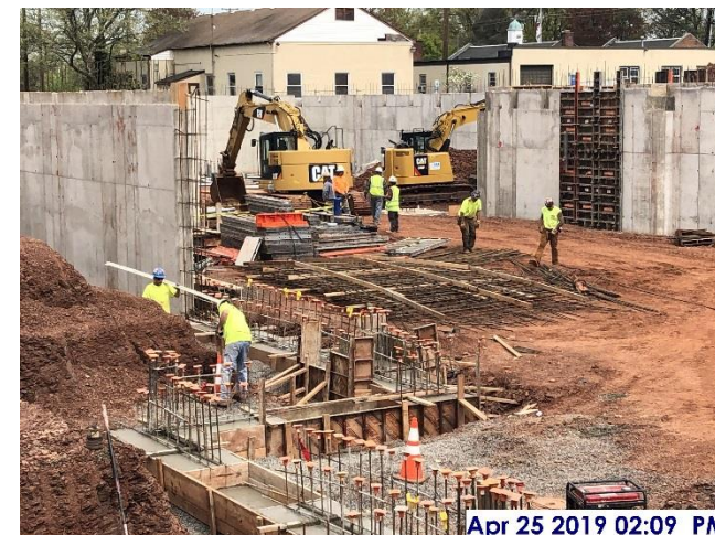
Apr 25 2019 02:09 PM Concrete for footing between center & west sectors
