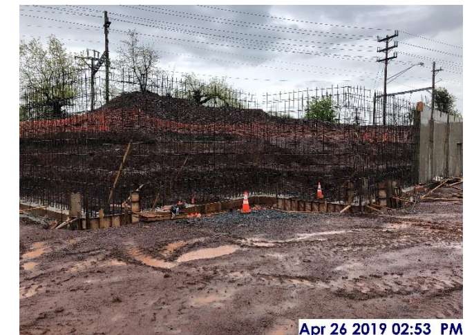
Apr 26 2019 02:53 PM Rebar for foundation wall between center & west sectors
