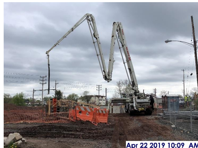
Apr 22 2019 10:09 AM Pumping concrete for south foundation wall, west sector
