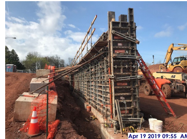
South Foundation Wall Formed in Western Section of Building
