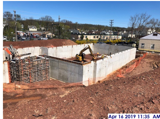
View of Eastside Foundation Walls
