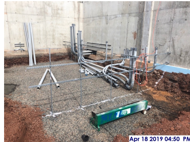
Under Slab Rough In of Electric Switchgear Room
