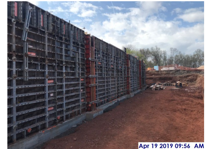
Another View of South Wall – Concrete Pour on Monday
