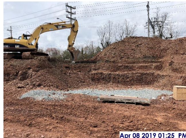
Excavation for north wall in western section
