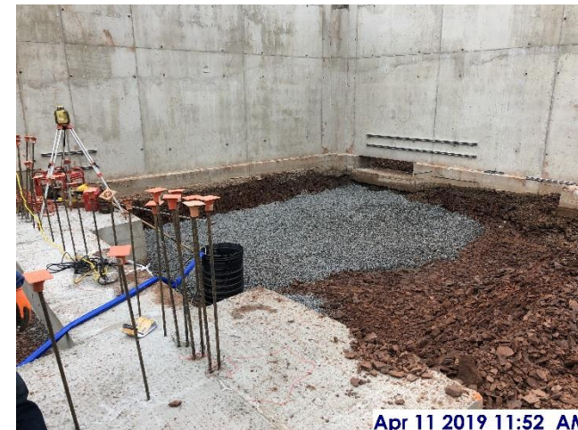
Stone placed for main electrical room in basement
