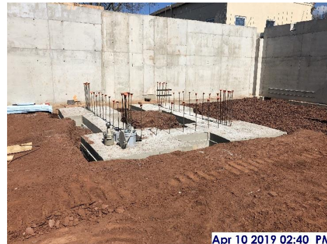
Stair tower footing
