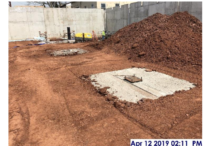
Interior piers backfilled and graded in eastern section
