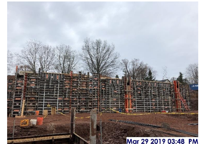
Closing form work for foundation wall, center sector
