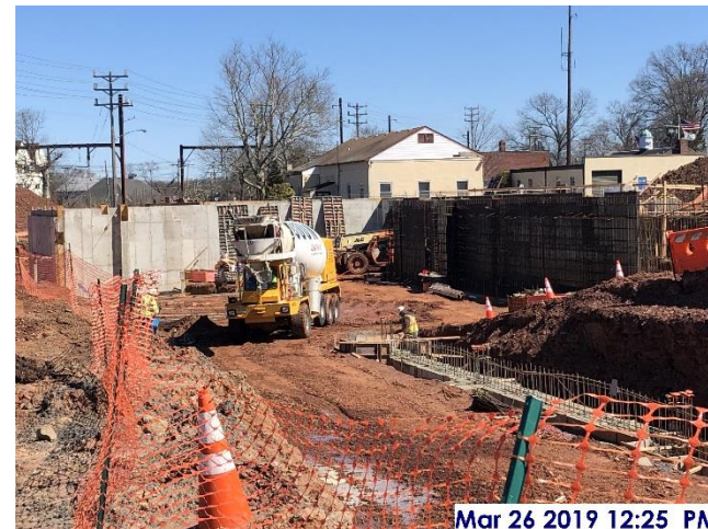
Pouring concrete for footings, west sector
