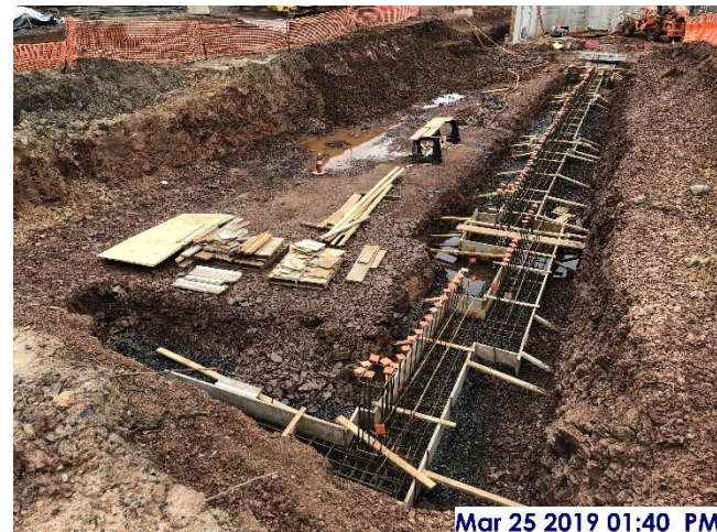
Form work and rebar for footings, west sector
