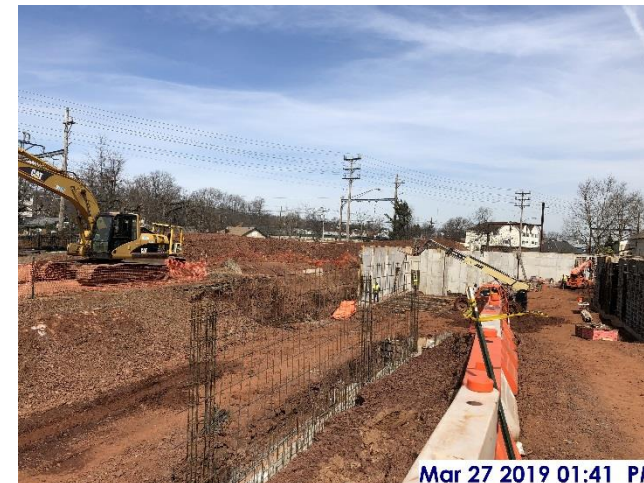
Starting rebar for foundation wall, west sector
