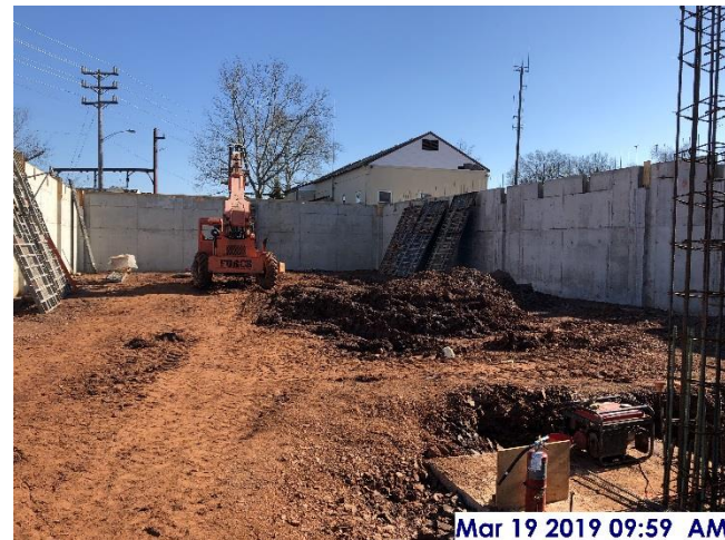
Foundation walls complete at southeast corner
