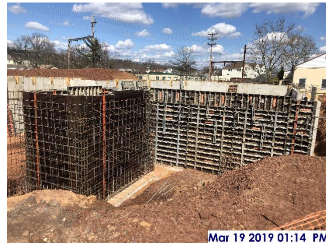
Form work for foundation walls at main entrance
