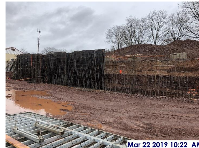
Rebar and form work for south foundation wall, center sector
