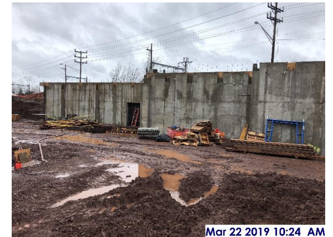
Form work stripped at north foundation walls
