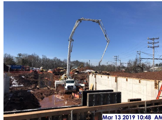
Pumping concrete for foundation walls
