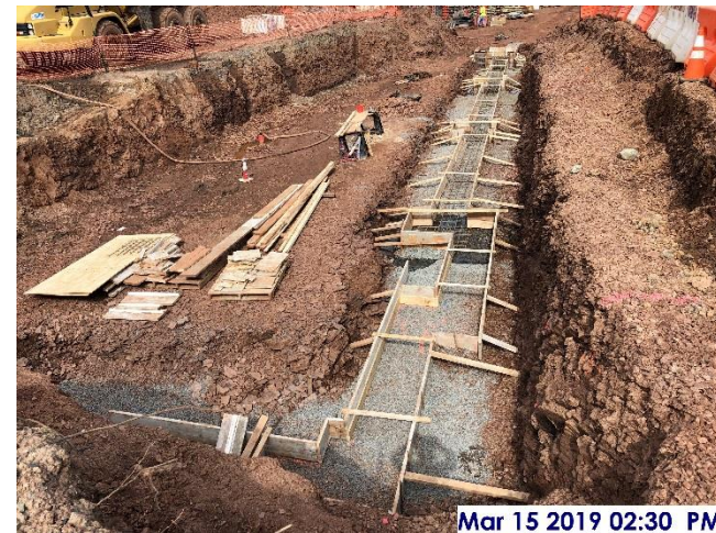
Form work for footings in west building sector
