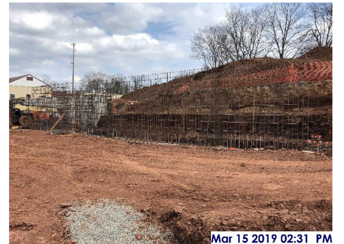
Rebar for south foundation wall in center building sector
