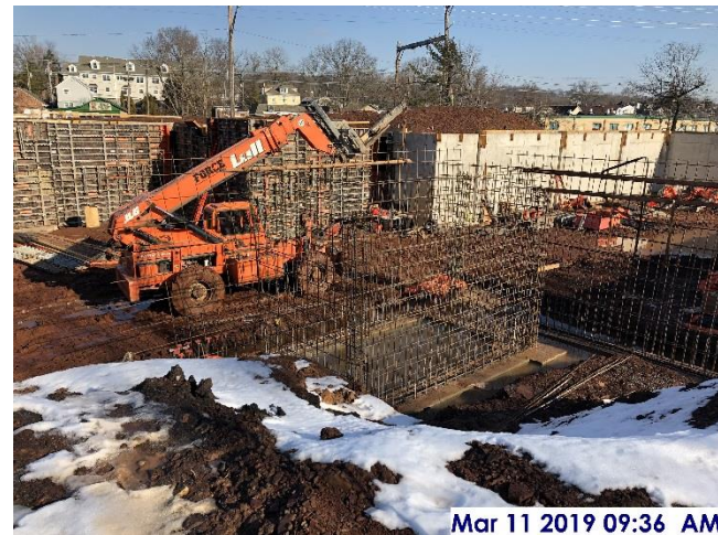
Rebar for foundation walls at main entrance
