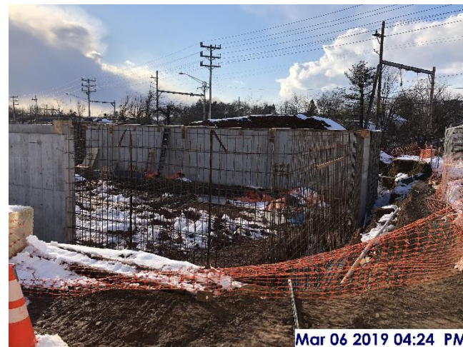
Rebar for foundation walls at southeast corner
