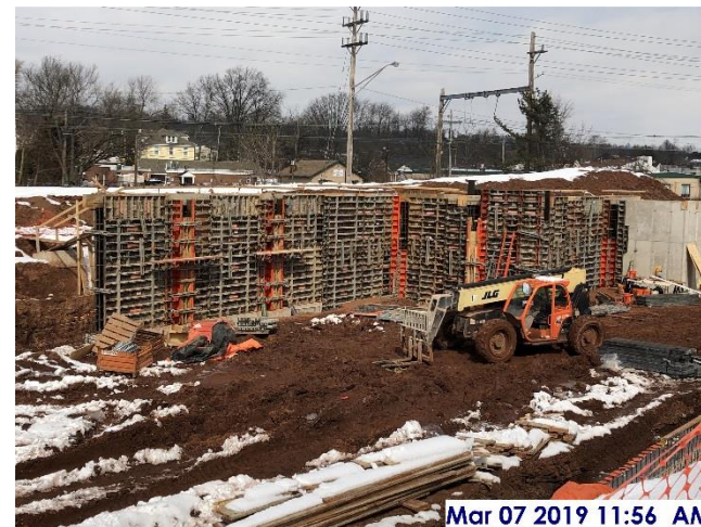
Closing up foundation walls on north side
