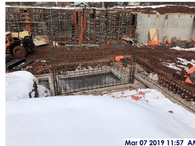
Foundation wall rebar at main entrance
