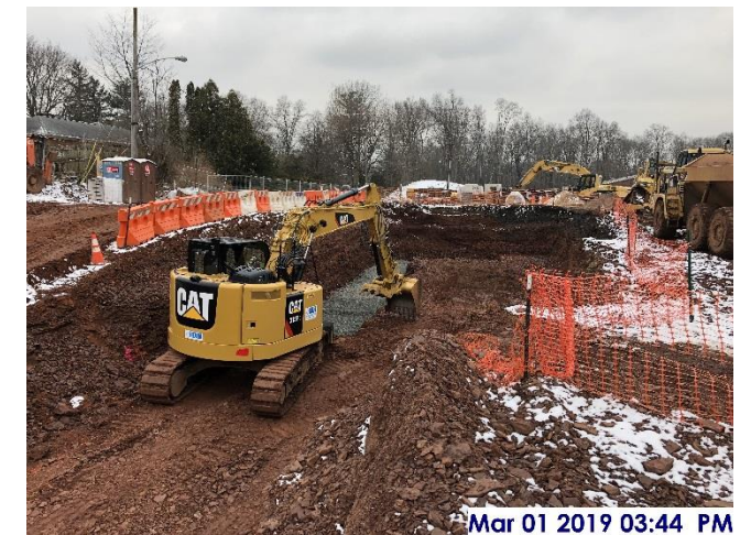
Basement excavation for west section of building
