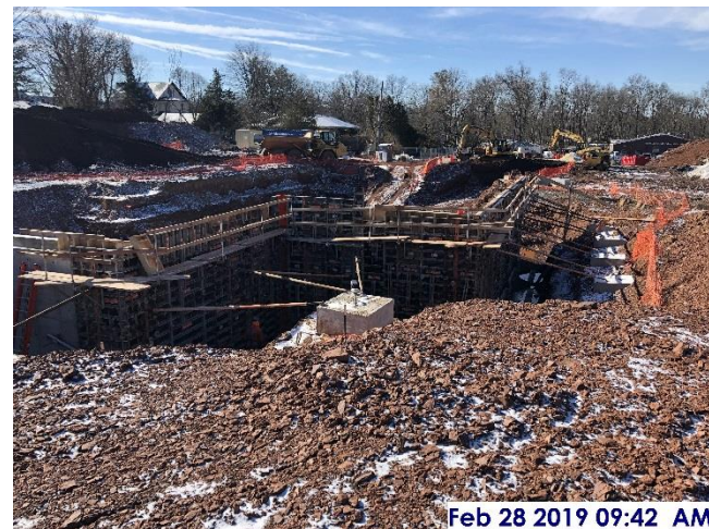
Form work and bracing for foundation walls
