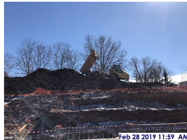
Stockpiling soil from excavations
