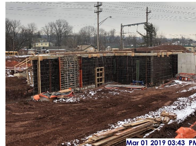
Rebar and form work for foundation walls
