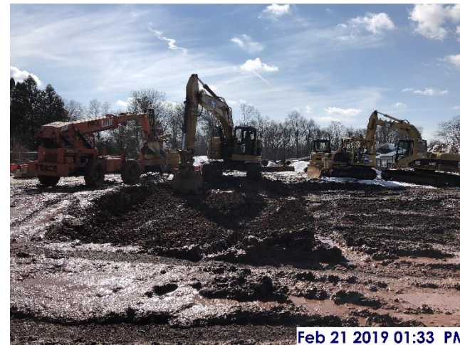
Beginning excavation for final third of basement
