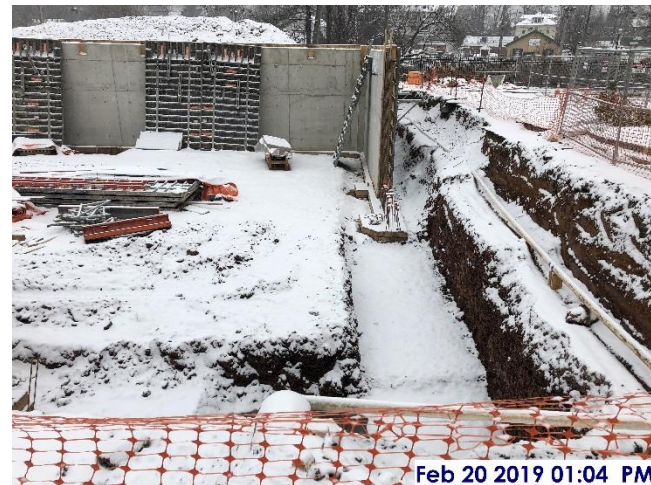
Continuing footing excavation at east end of building
