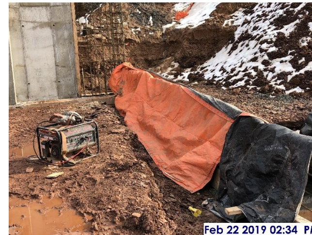
Blanketed concrete footing near future front entrance
