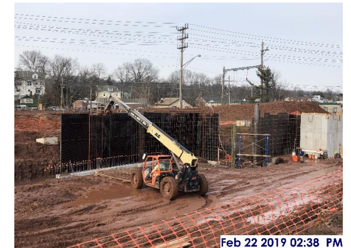
Rebar and form work for foundation wall at building rear
