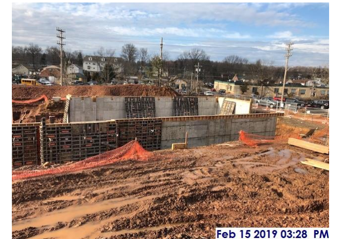
Stripping form work from foundation walls
