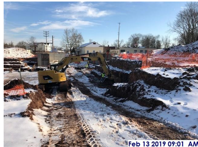
Excavation for footings
