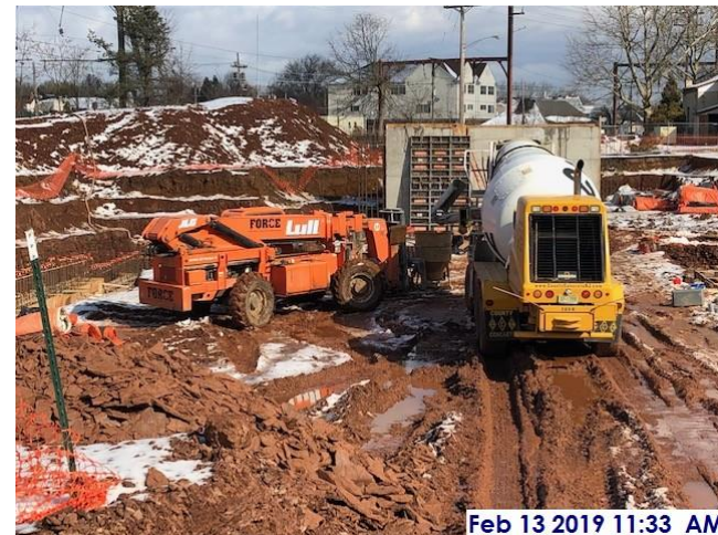
Pouring concrete for footings
