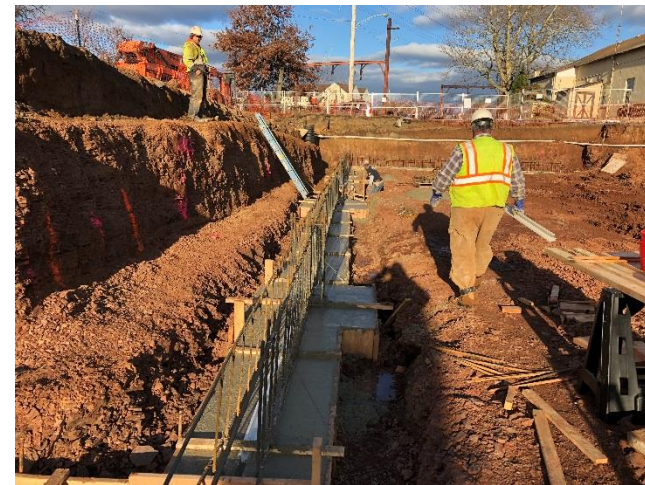
First concrete poured for new Municipal Building foundation
