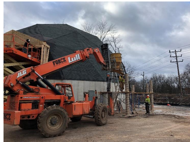
Pouring concrete for salt dome brine tank shed piers
