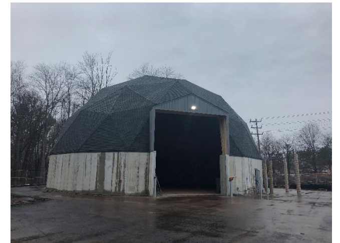
Main salt dome structure substantially complete
