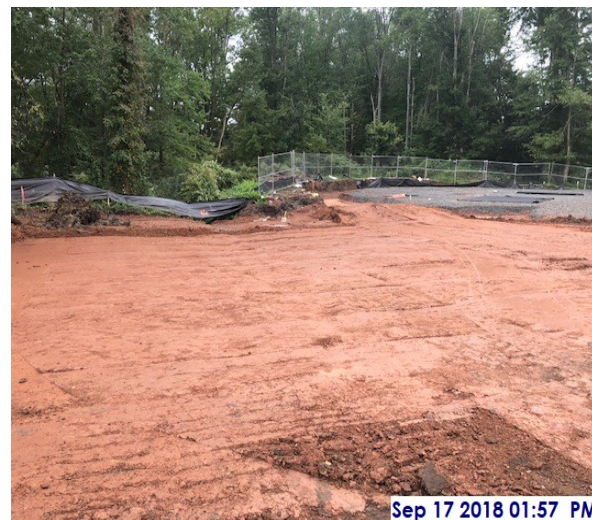
Proofrolled area near the new Salt Dome
