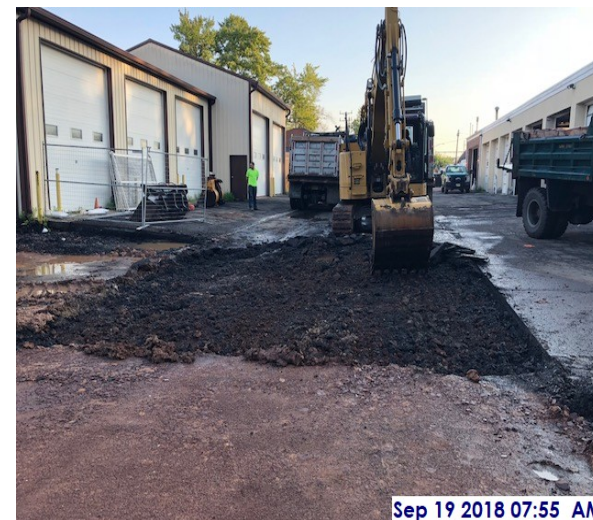
Asphalt being excavated near the DPW Garage
