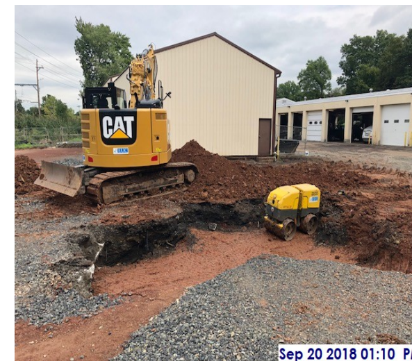
Soil being compacted near the new Salt Dome
