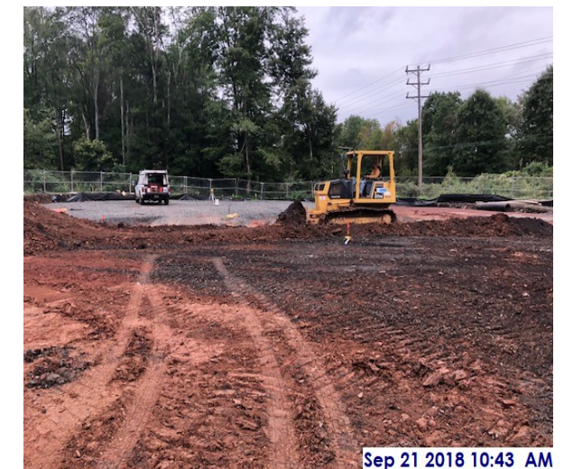
Regrading of soil near the new Salt Dome
