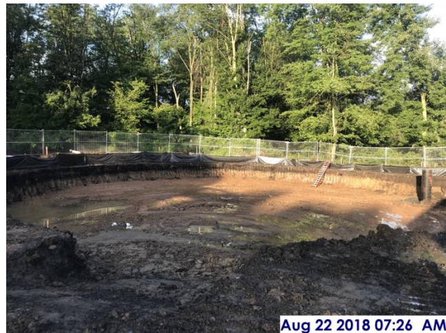
Excavation to subgrade at New Salt Dome
