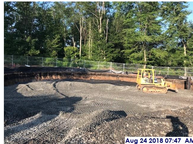
Stone being spread at New Salt Dome Area
