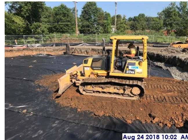
Backfilling at New Salt Dome
