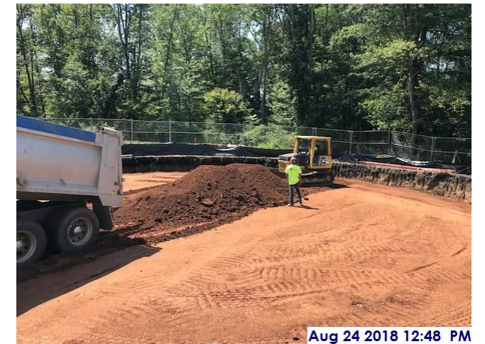
1 st backfill lift completed. 2 nd lift started
