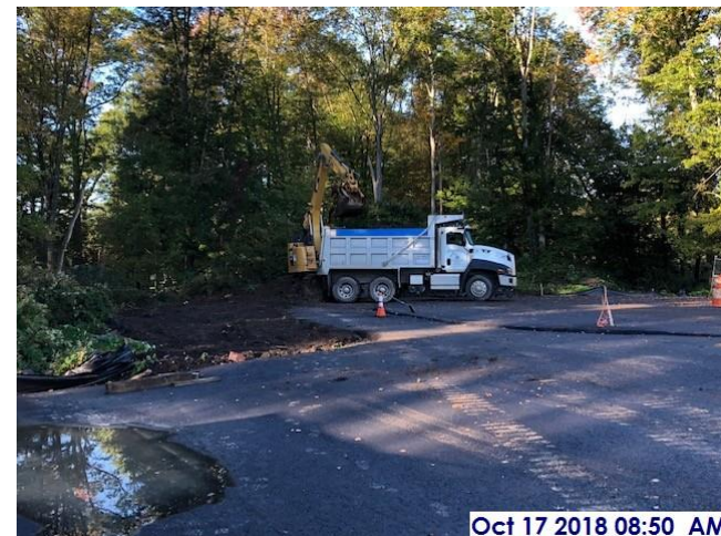
Shaving soil berm behind new salt dome site
