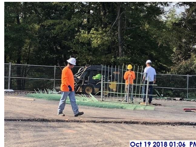
Preparing rebar for new salt dome
