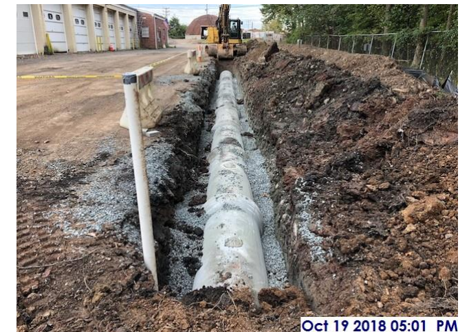
Concrete pipe and stone fill for storm line
