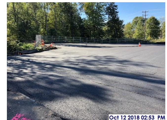
Asphalt base layer at new salt dome site
