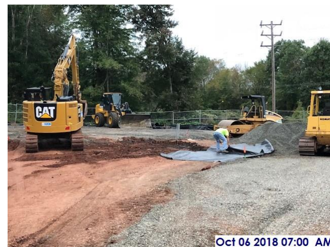
Installing fabric and DGA at new salt dome site
