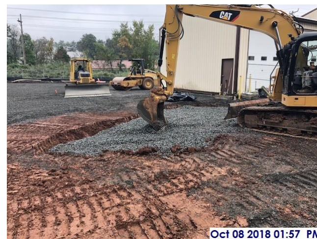
1.5" stone installed at entrance to new salt dome site
