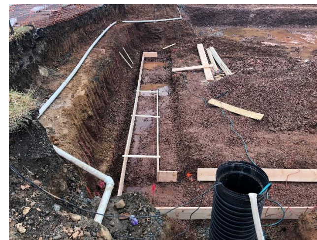
Beginning form work for Municipal Building foundation
