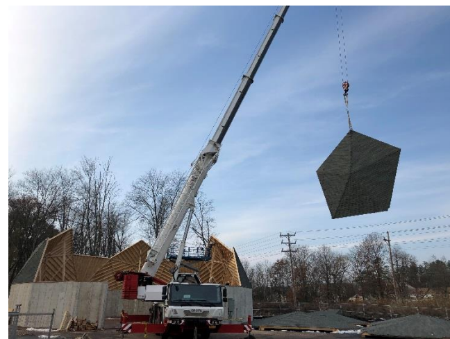
Lifting salt dome panel
