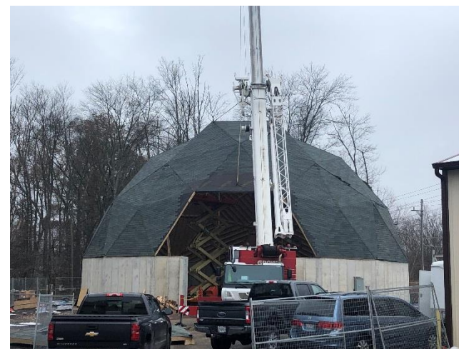
Setting front salt dome panel over entrance
