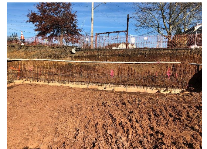
Rebar for Municipal Building foundation
