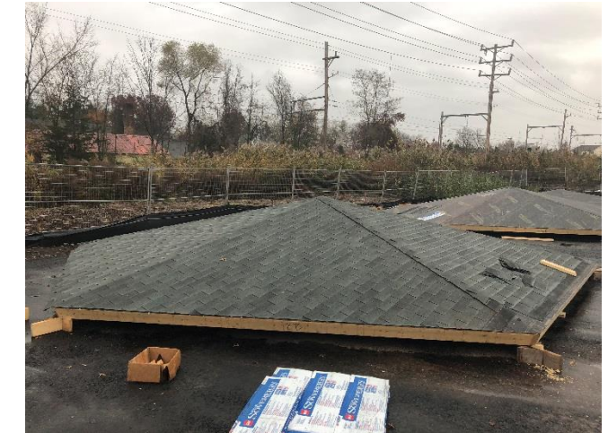
Shingling of salt dome panels
