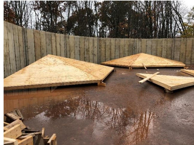
Salt dome panels under construction
