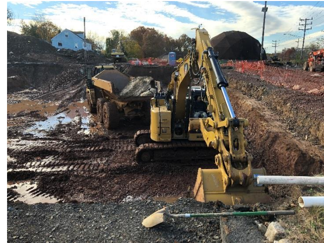
Additional basement excavation for Municipal Building
