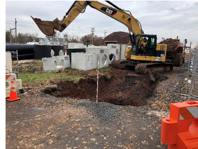
Excavation for storm inlet at Columbus & Berkeley Aves.
