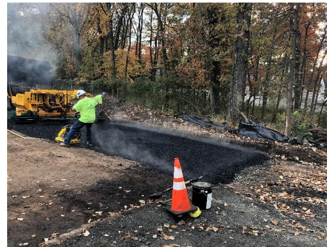
Spreading asphalt at new DPW storm and water lines
