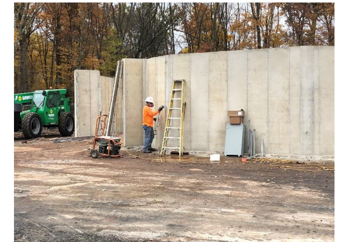
Finishing concrete at new salt dome walls
