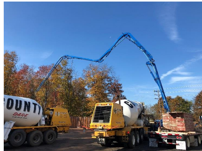
Pumping concrete for new salt dome walls
