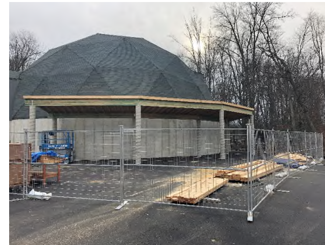
Framing for brine tank storage shed
