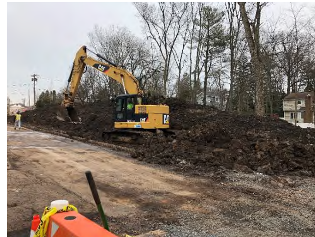
Berm construction continuing in DPW area
