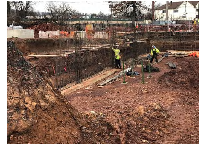
Rebar for Municipal Building foundation walls & columns
