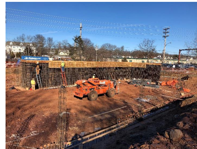
Form work for foundation walls
