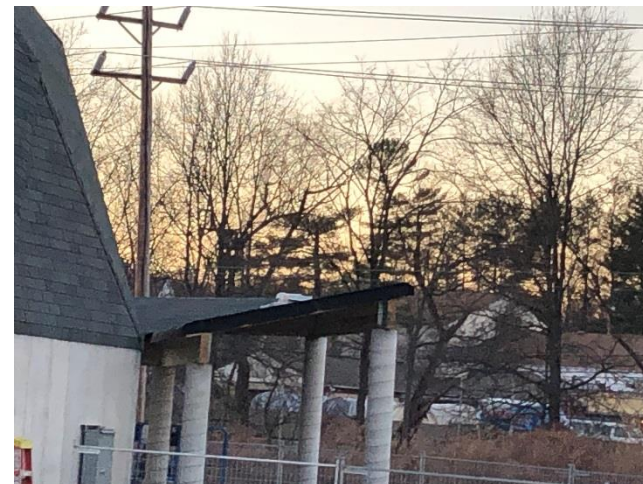
Roofing for brine tank storage shed
