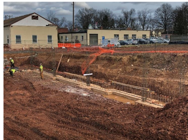
Rebar for foundation walls and columns
